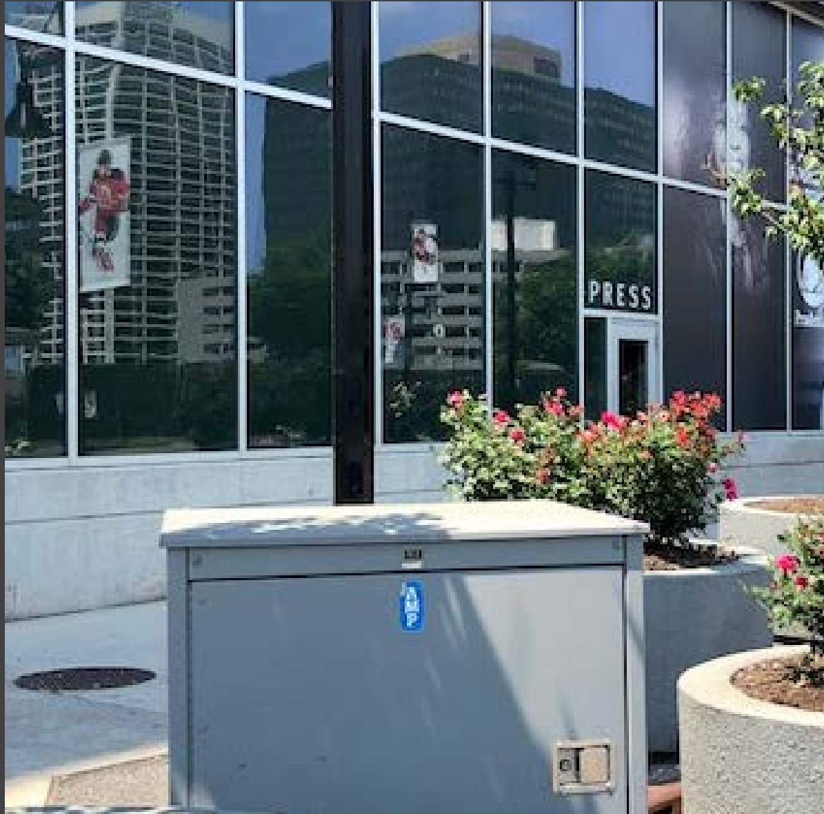
Mulberry Street Pedestal (if cooking outside) One 200A/3 Phase; 208Y/120V
